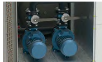
Pump section with or without storage tank.
